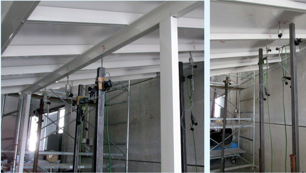
Photos of veranda showing displacement transducer arrangement on the underside
