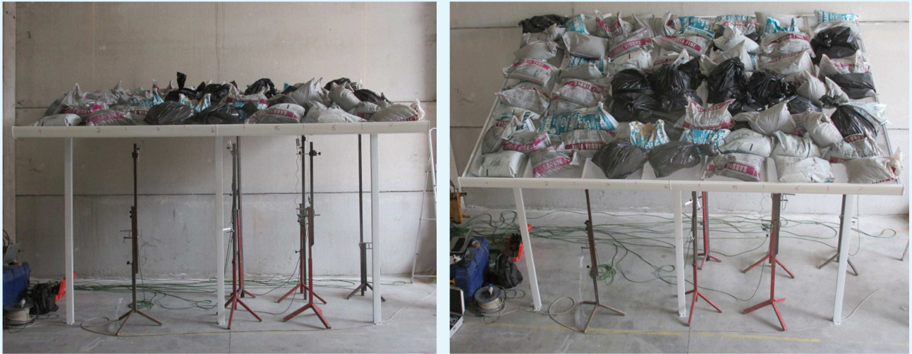
Photos of veranda showing sandbag distribution during maximum load step 5
